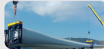
Blade lifting at port
