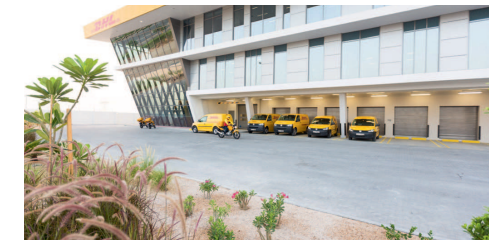
OPEN FOR DELIVERY: New facilities will provide increased efficiency.
